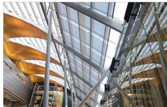
Tension Shading System in atrium and Dynamic Facade Control System - Darling Quarter, Sydney.
