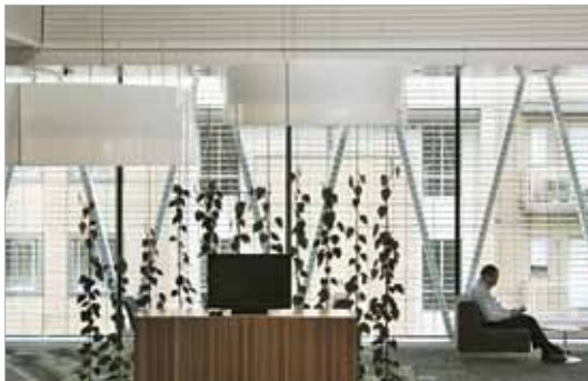
Speciality Venetian Blinds in double skin facade and Dynamic Facade Control System - NZI, Auckland, New Zealand.
