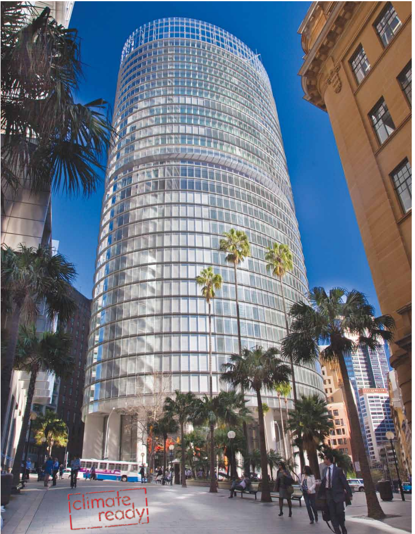
No 1 Bligh Street - Complex geometry raises solar control delivery External Venetian Blinds integrated with fully automated control
