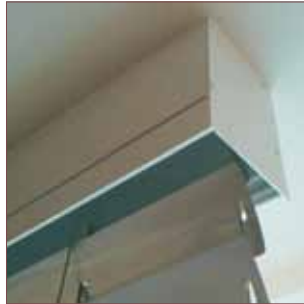
Aluminium skirting detail with 50mm extension
